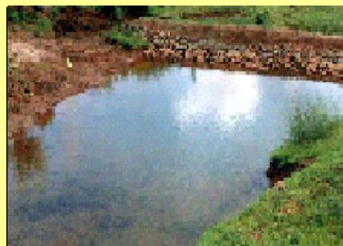
Earthen gully plug
