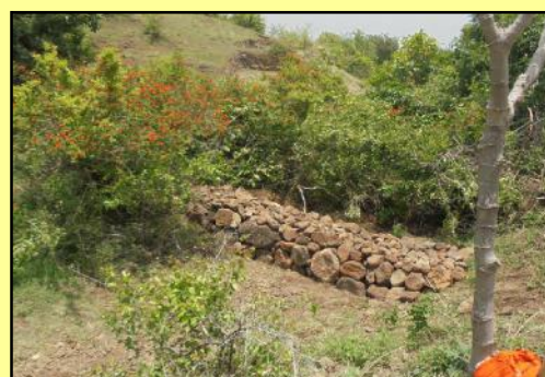
Completed gully plug
