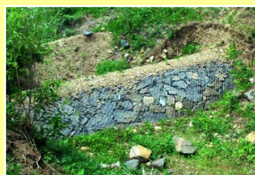
Gabion structure
