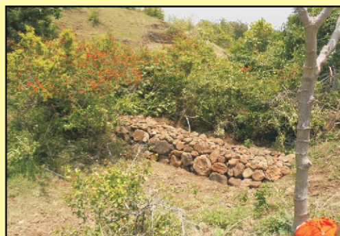
Completed gully plug
