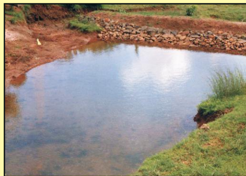
Earthen gully plug
