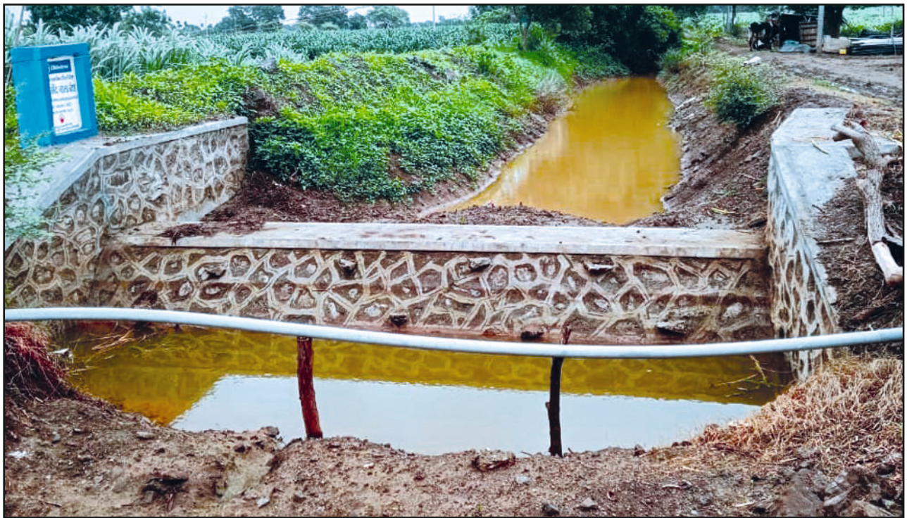
Cement nala bund construction
