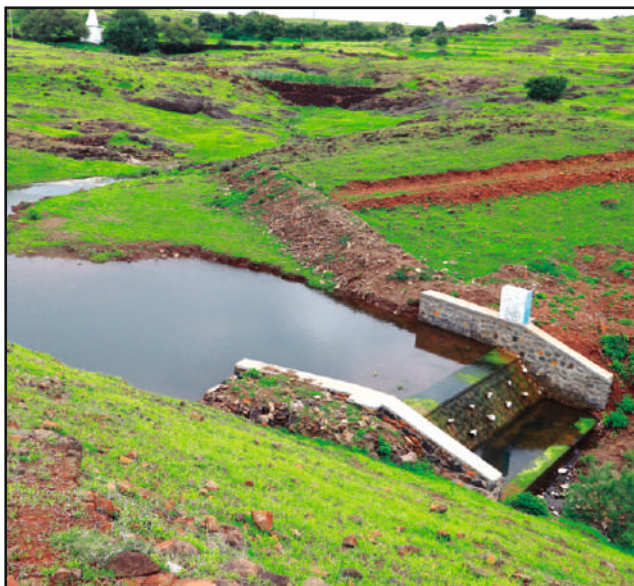
Construction of cement nala bunds
