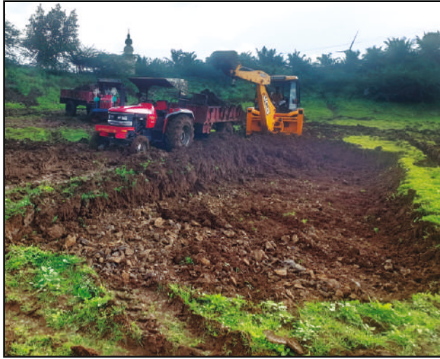
De-siltation of percolation tank
