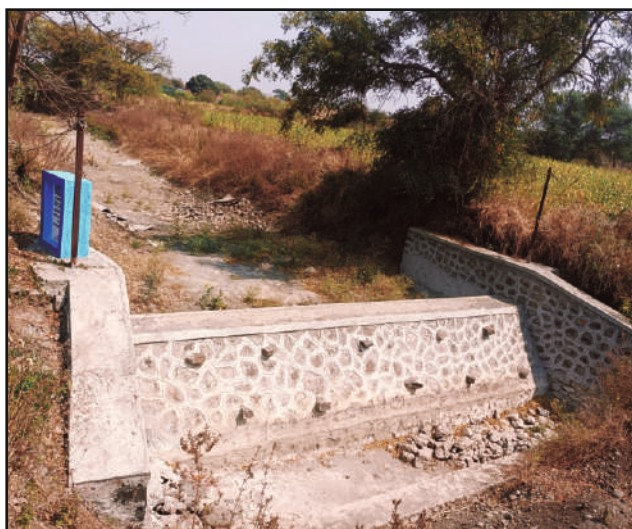
New cement nala bund construction
