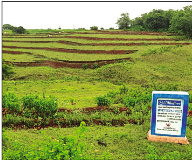
Continuous Contour Trenches
