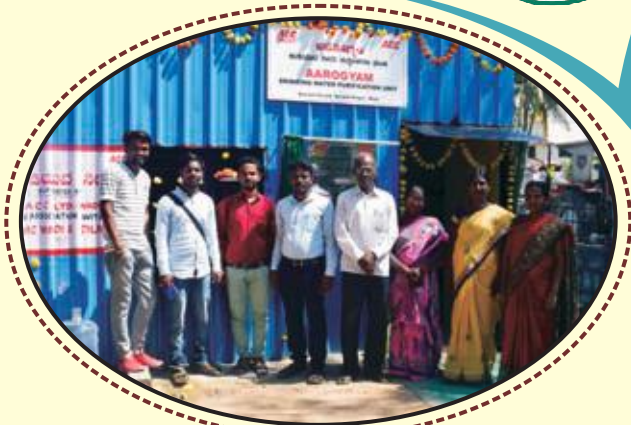
Community RO Water Plant
