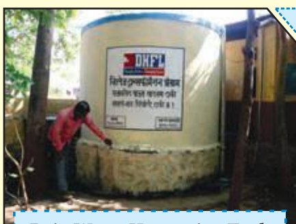
Rain Water Harvesting Tank
