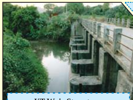
KT Weir Structure
