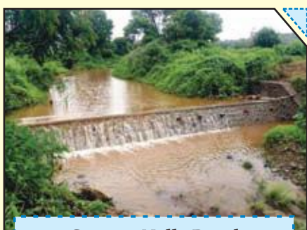
Cement Nalla Bund
