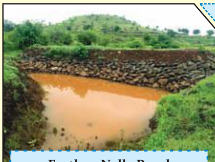
Earthen Nalla Bund
