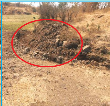
New Drainage Channel to Field
