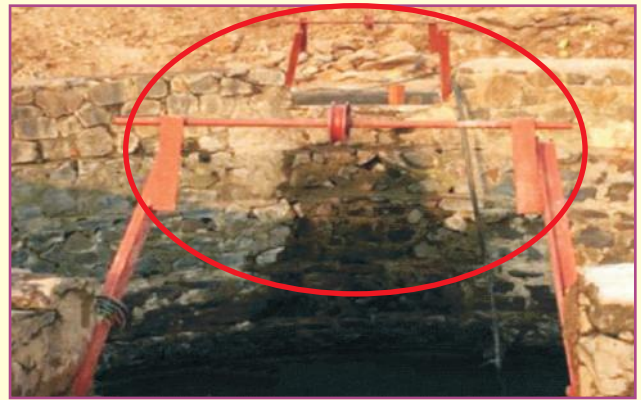
Installed new Pulleys
